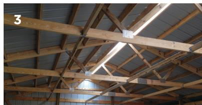
**3) Truss to truss bottom chord bracing:** Roof trusses must be straight and plumb to support their design loads. Bottom chord bracing maintains truss alignment under high wind loads. Special connection hardware ensures the bottom chord braces are effective in both compression and tension thereby providing positive reliable truss bracing.
