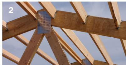
**2) Purlin to truss connection:** Purlins in steel hangers provide positive truss bracing (the truss cannot prematurely buckle) and eliminates places for birds to nest versus purlins above the truss.
