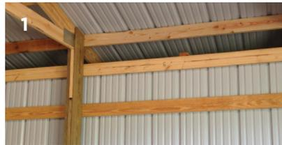
**1) Truss to column connection:** A symmetrical truss centered on the column eliminates an unexpected load on the column. It minimizes the risk of the column bowing. With a side mounted truss connection a large torque can be produced that could cause the column to bow, reducing the column's ability to carry its vertical load.
